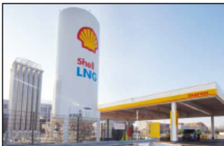
Europe's LNG refueling network is expanding – a station in Rotterdam.
