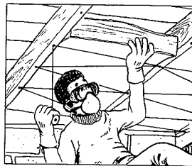
LACING WIRES ON NAILS SET INTO JOISTS
